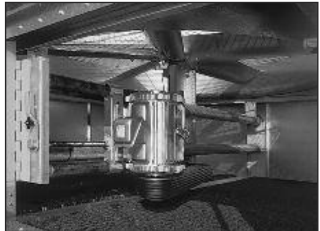
Motor Base Assembly
